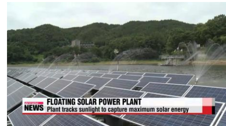
3MW floating photovoltaic power plant on Otae Reservoir, Sangju City, Gyeongsang Bukdo Province
