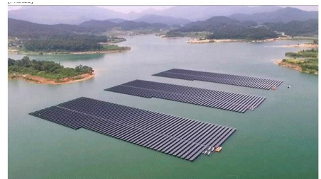
3MW floating photovoltaic power plant on Otae Reservoir, Sangju City, Gyeongsang Bukdo Province
